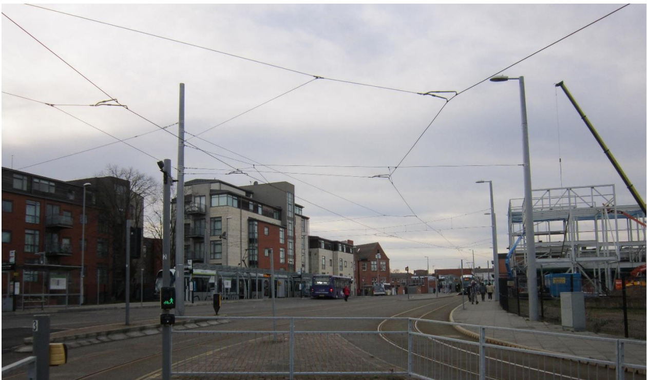
Styring Street – Manor Centre development and transport interchange
